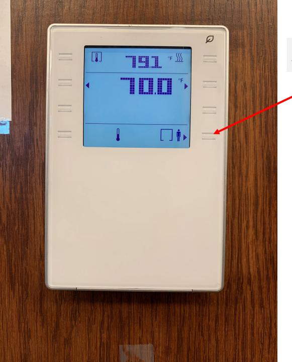
Now that the screen is "lit", push this button for 4 hours of cooling
