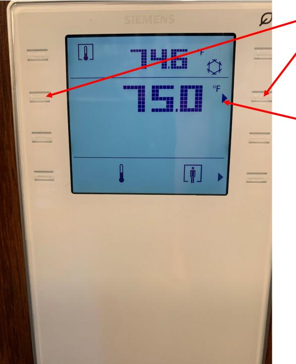
You can then adjust the room set point up or down by pushing these buttons.
